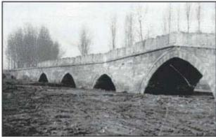
Its decorative bond is characterised by alteration of reddish and greyish ashlars. It is asymmetrical, and the span of its central arch reaches about 13m. It is more than 135 m long, and has almost 5 m in width.
